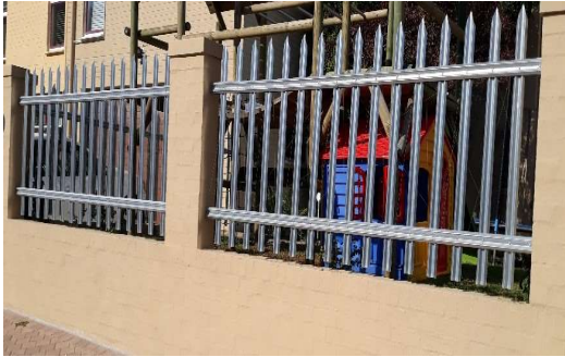
Specification 16: Palisade Fence 2
