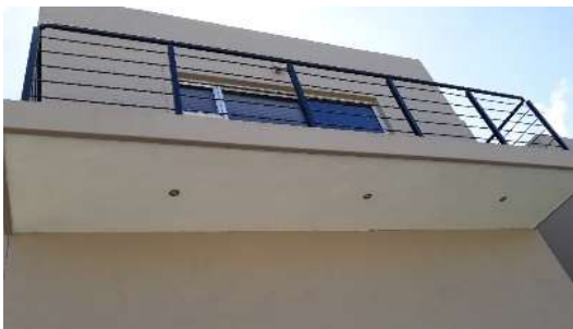
Specification 12: Balustrade/ Hand rail 4
