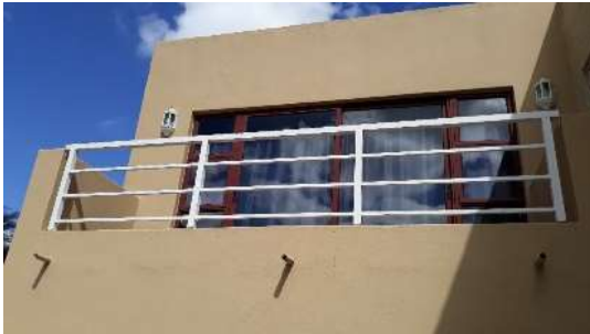
Specification 10: Balustrade/ Hand Rail 2
