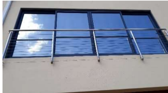
Specification 11: Balustrade/ Hand Rail 3
