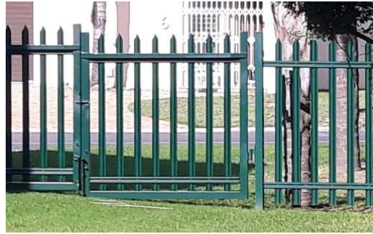
Specification 17: Palisade Fence 3
