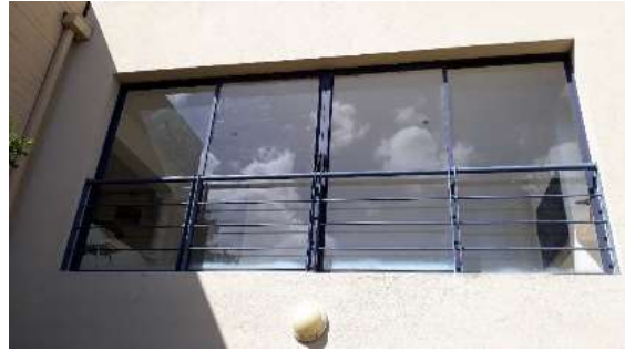
Specification 9: Balustrade/ Hand Rail 1
